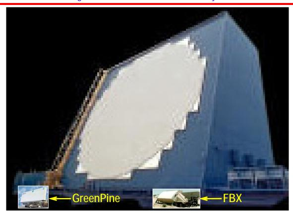
National Missile Defense Ground-Based Radar Prototype (NMD-GBR-P) X-Band Radar to be Used in National Missile Defense System
